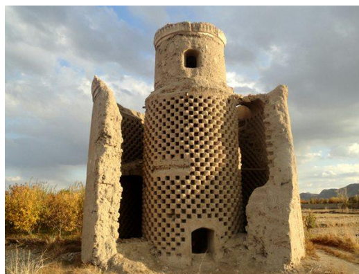
Picture (4): Remains of one of the pigeon tower, shows the inner and outer tower's drums
